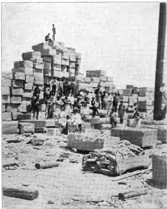
MATERIAL READY FOR SHIPMENT, BEALER QUARRY
